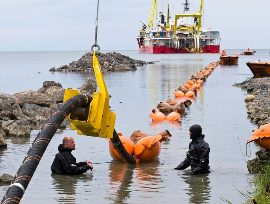
Figure 3-6. The photo shows the pull-in to shore of bundled cables, where the fibre optical cable is strapped to the power cable. A fibre optic cable is visible on the left side of the power cable.
