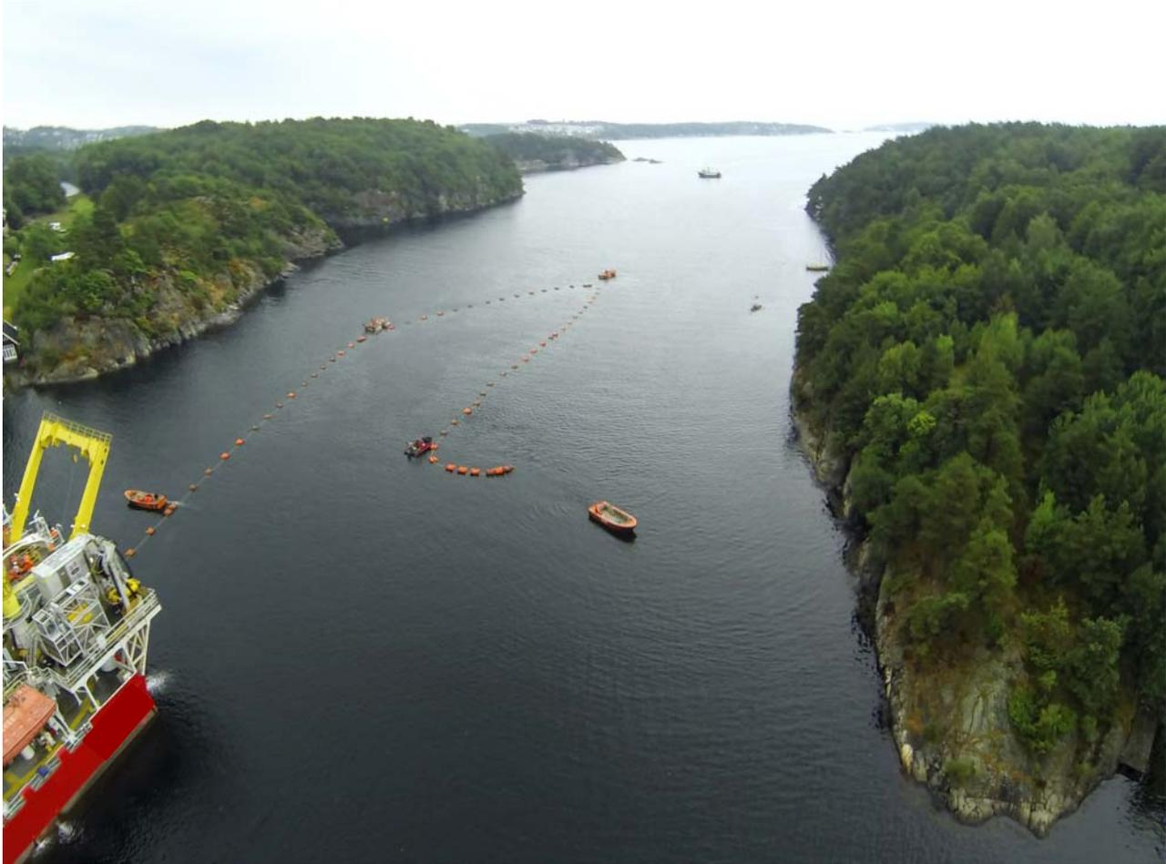
Figure 3-3. Submarine cable carried on floats from the cable laying vessel to shore.
