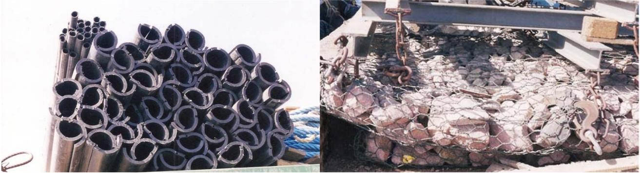
Figure 3-12. Left: split PE pipes ready for fitting around cable prior to covering with the cobble-filled gabion mattresses in a sub-tidal area with a hard seabed material. Right: cobble-filled gabion mattresses ready for placing over split PE pipes.
