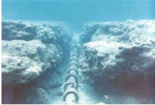
Figure 3-13. Split-pipe articulated cable protectors installed on cables placed in a trench.
